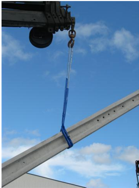
Erecting with a safety bolt and polyester or composite material sling stop
