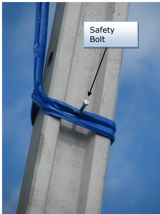
Erecting with a safety bolt and polyester or composite material sling stop
